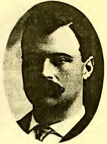
JOHN J. OWENS, Railway Conductor.
