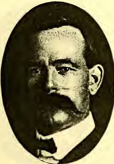
JAMES ALBERT SMITH, Contractor, Lisbon, Ohio.
