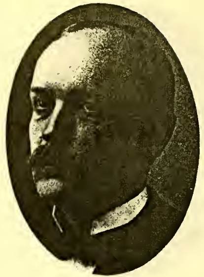
JOHN H. HALL, Moulder. Deming Pump Works.
